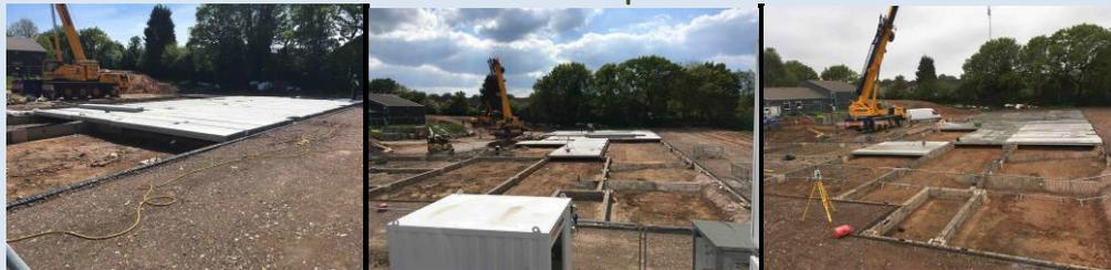
ISG have installed the sub-station base and began the installation of the pre-cast ground floor slab. Keep watching the progress made each week on our twitter web page.
